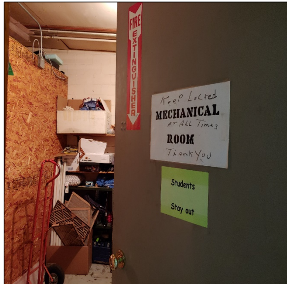
Unlocked Maintenance Closet*
