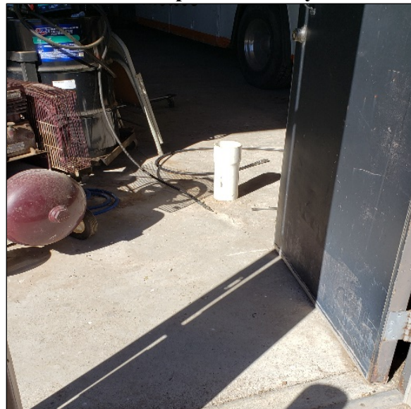
PVC Pipe in Doorway
