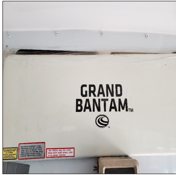
Repair Made With Packing Tape
